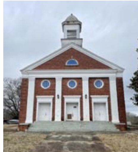
View of outside the church
