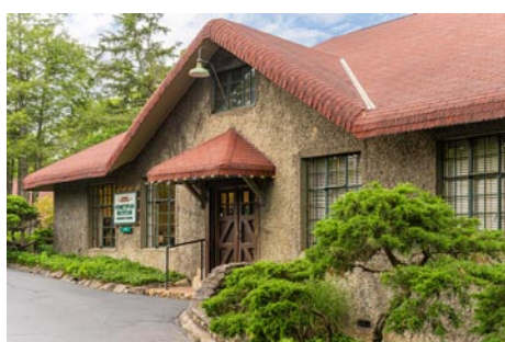
View of one of the Grovewood Village Buildings
