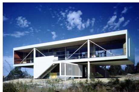
The Julian Rose House, Design/Completion 1949-1950, Wahroonga, Sydney, Australia, Steel structure, timber infill
